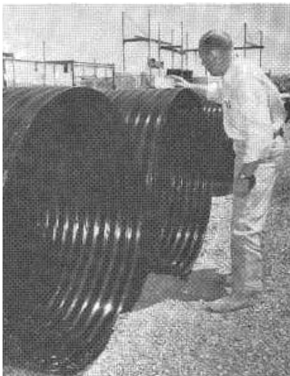
Bituminous-coated corrugated metal pipe is inspected .
