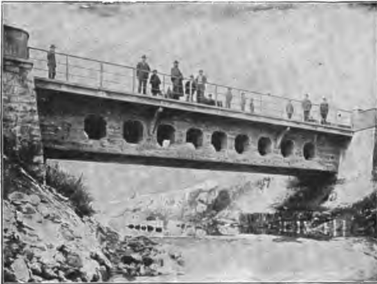
FIG. 277.—Bridge near Krapina, with open girders of 200 m. (66 ft.) span.
