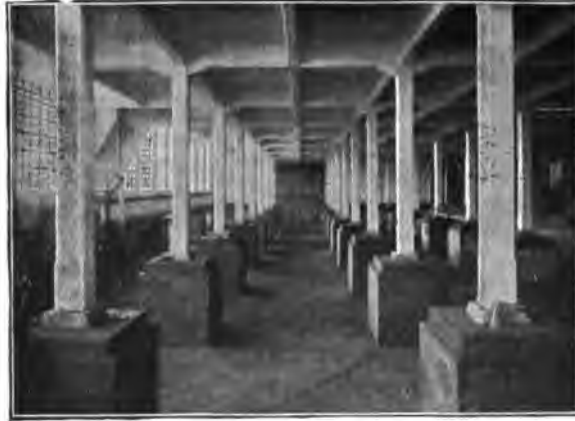
FIG. 260.—Woven wire reinforcement for a water-tight cellar in reconstruction of the Daimler motor factory in Unterturkheim.
