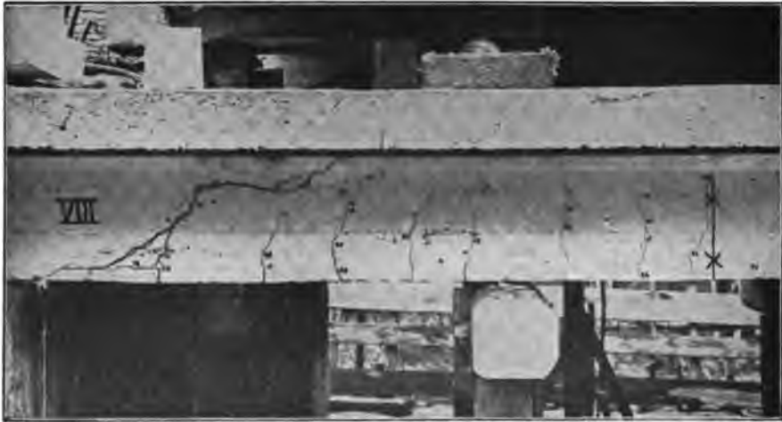
FIG. 155.—Beam VIII, under the breaking load.
