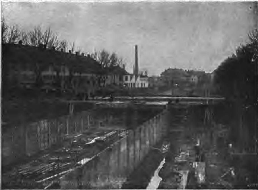
FIG. 287.—Cover of the Ill-Hochwasser Canal, Mülhausen.
