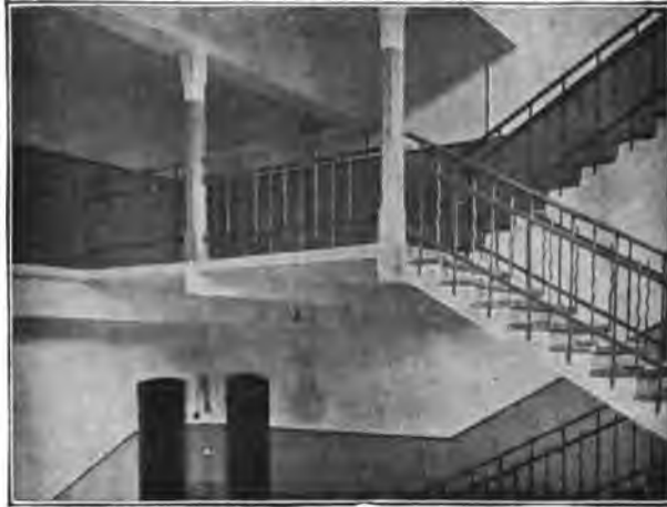
FIG. 242.—Reinforced concrete stairs with suspended platforms in the brewery in the English Garden in Stuttgart.
