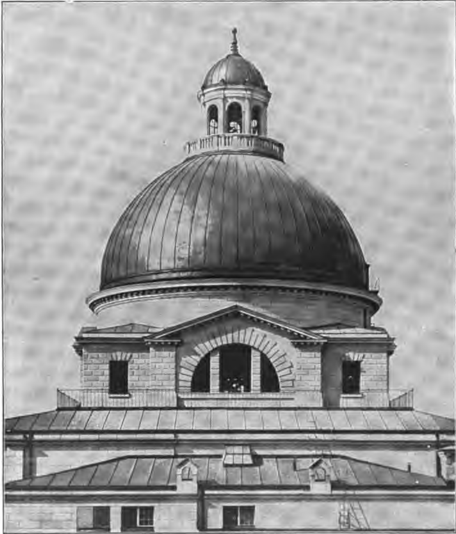
FIG. 250—Reinforced concrete cupola and lantern of the Army Museum in München, diameter 36 m. (52.5 ft.).
