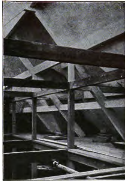
FIG. 232.—Reinforced concrete roof supports in the building of the “Münchener Neuesten Nachrichten.”
