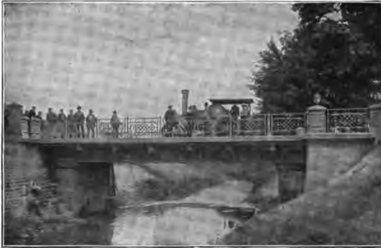
FIG. 275.—Hornback Bridge near Zweibrücken.
