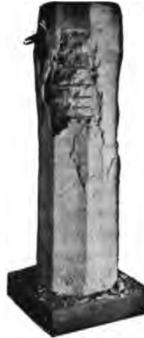
FIG. 73.—Spalling of the outer concrete shell.
