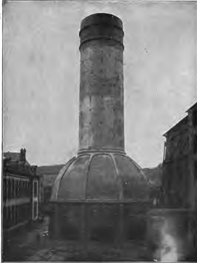
FIG. 346.—Cooling tower of the Differdingen Steel Works.
