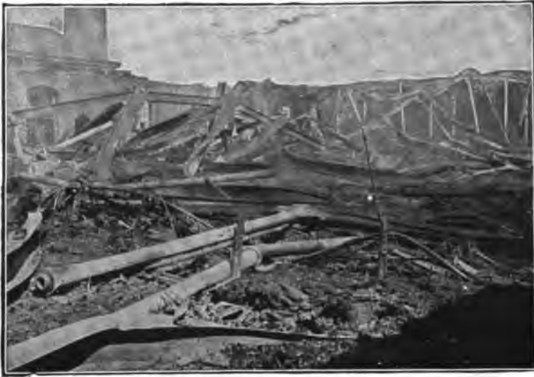
FIG. 203.—Top Floor of the Speyer Cotton Mill after a Fire.
