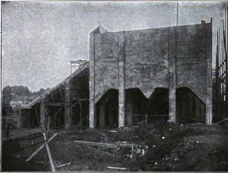
FIG. 332.—Maizière ore pockets. 178 m. (583 ft.) long.
