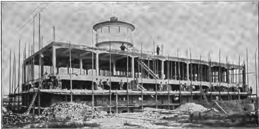
FIG. 202.—Warehouse for the Government Railway at Elberfeld in Opliden.
