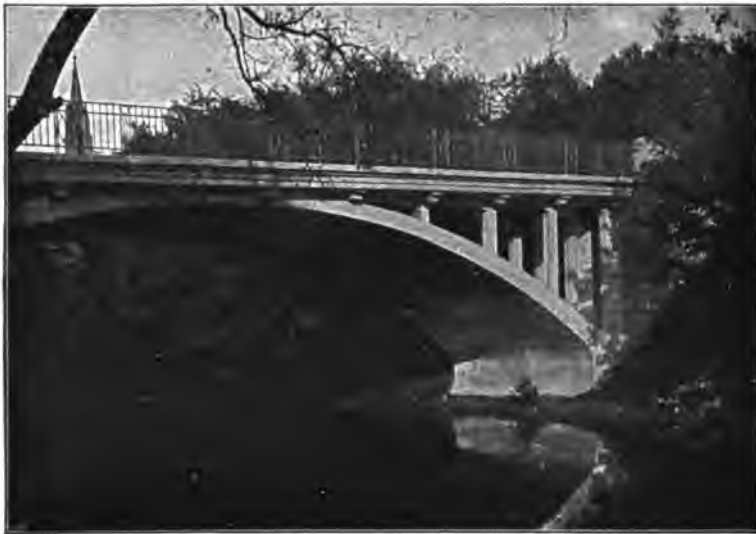
FIG. 305.—Nagold Bridge near Caln (Württemberg).
