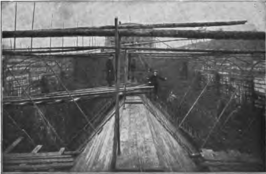
FIG. 337.—Düdelingen ore pockets. Placing reinforcement.
