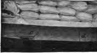
FIG. 170.—Bursting effect of loose diagonal stirrups.
