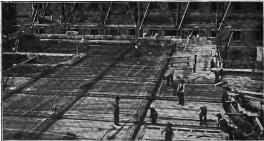
FIG. 224.—Placing reinforcement for Tietz shop.
