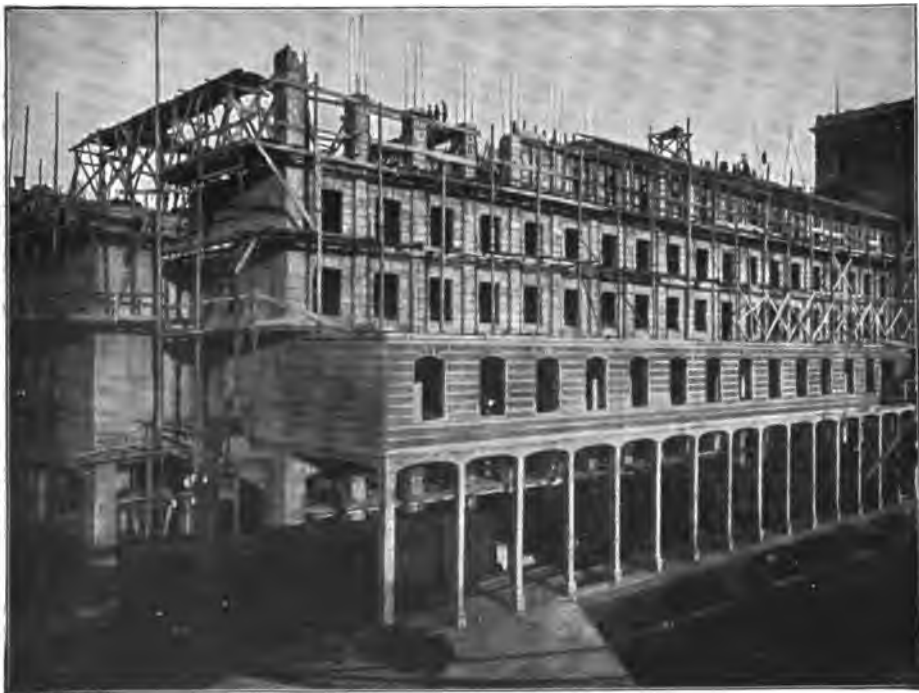
FIG. 341.—View of the silo in Genoa with the colonnade toward the harbor.
