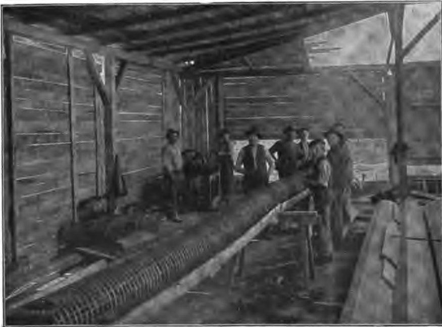
FIG. 265.—Factory in Metz. Fabrication of pile reinforcement.
