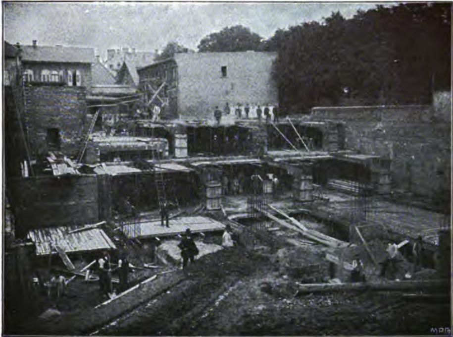
FIG. 227.—Erection of the three-story Deinhardt wine cellar, Coblenz.
