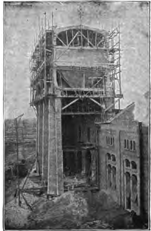
FIG. 324.—Sawdust bins of the Waldhof Pulp Mill.
