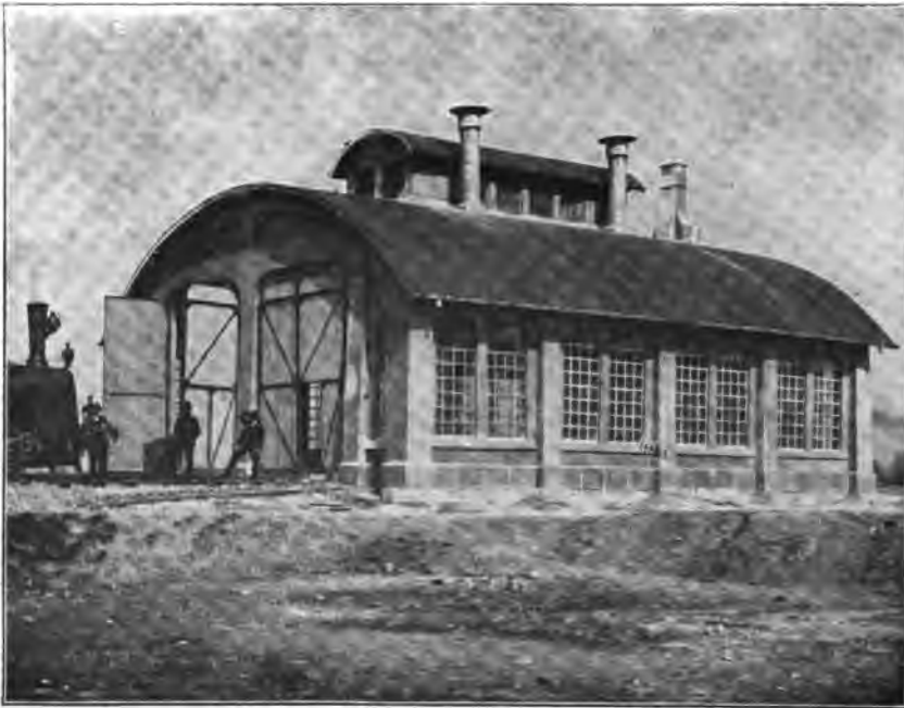
FIG. 237.—Exterior view of locomotive house in Krefeld.
