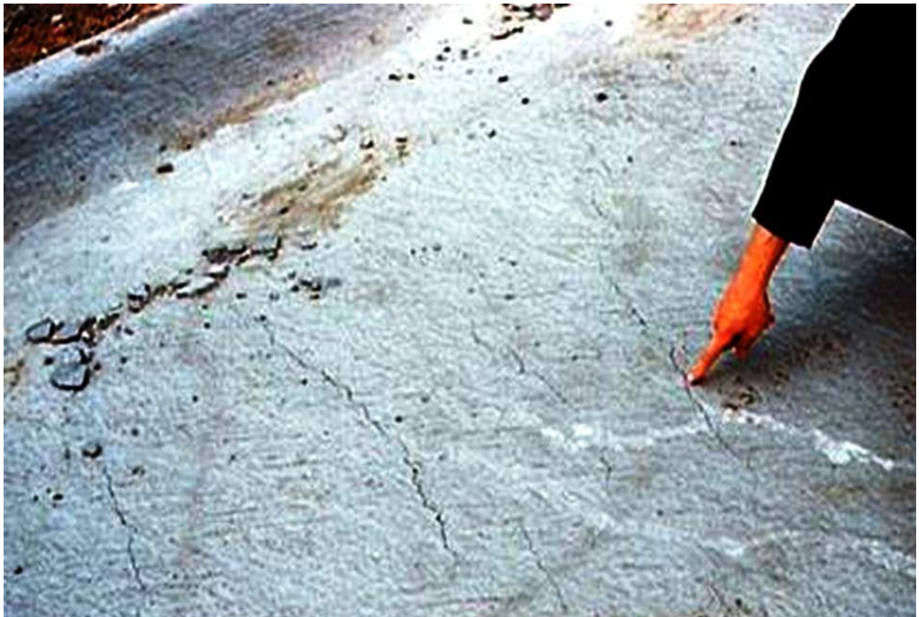
Fig. 13-7. Typical plastic shrinkage cracks. (IMG12267) Design and Control of Concrete Mixtures - Steven H. Kosmatka
