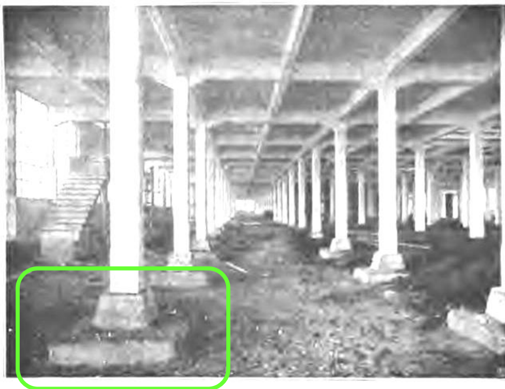
FIG. 212.—Foundations, Daimler motor factory near Stuttgart.
