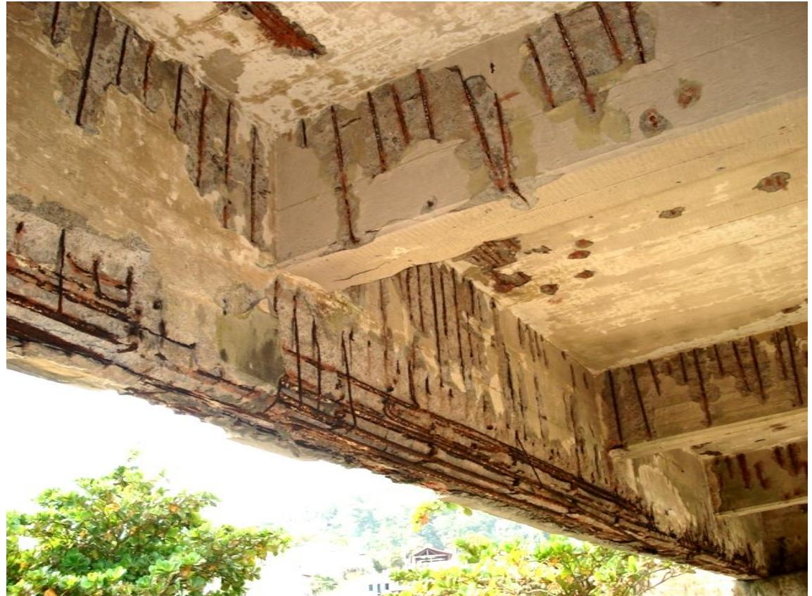
**Similarly, Dechamps et al., who carried out a programme of coring of actual structures to investigate corrosion at cracks, found that very little corrosion occurred where cracks crossed bars but the transverse bars (ESTRIBOS) were considerably more heavily attacked.**
