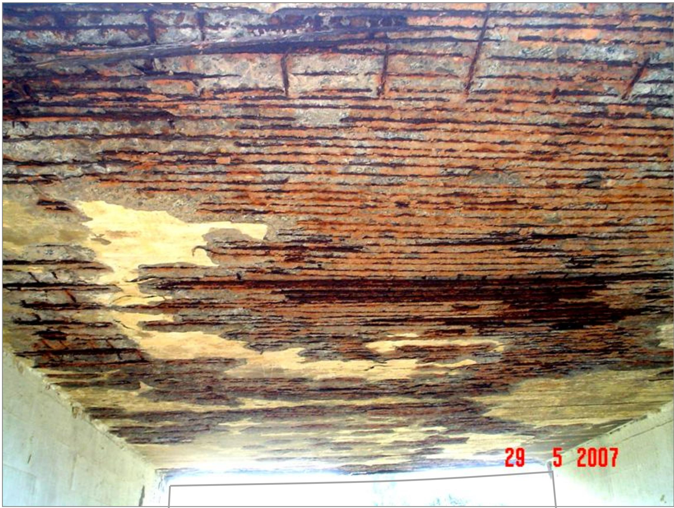
**EXEMPLO DE CORROSÃO EM ARMADURA DE LAJE EM ANTIGA PONTE NA RESTINGA DA MARAMBAIA / RJ**
