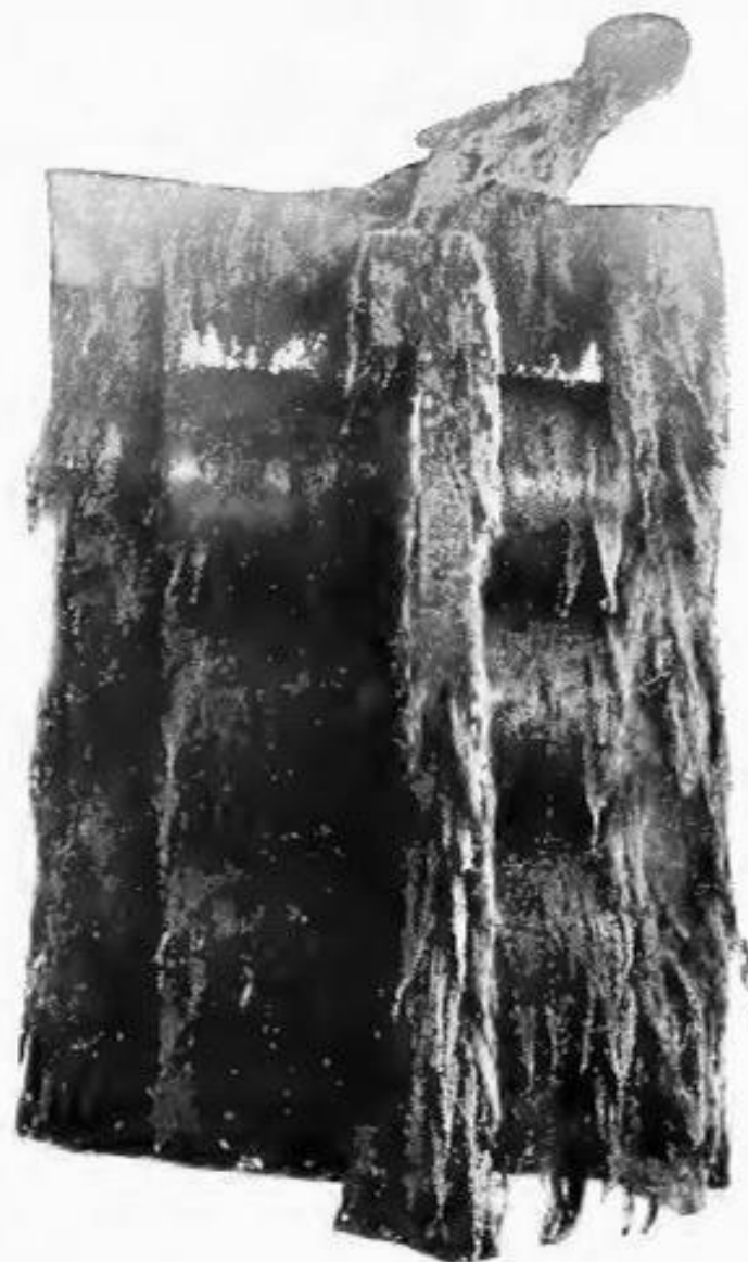
Fig. 20.— Crate with concrete test pieces after storage in sea water
