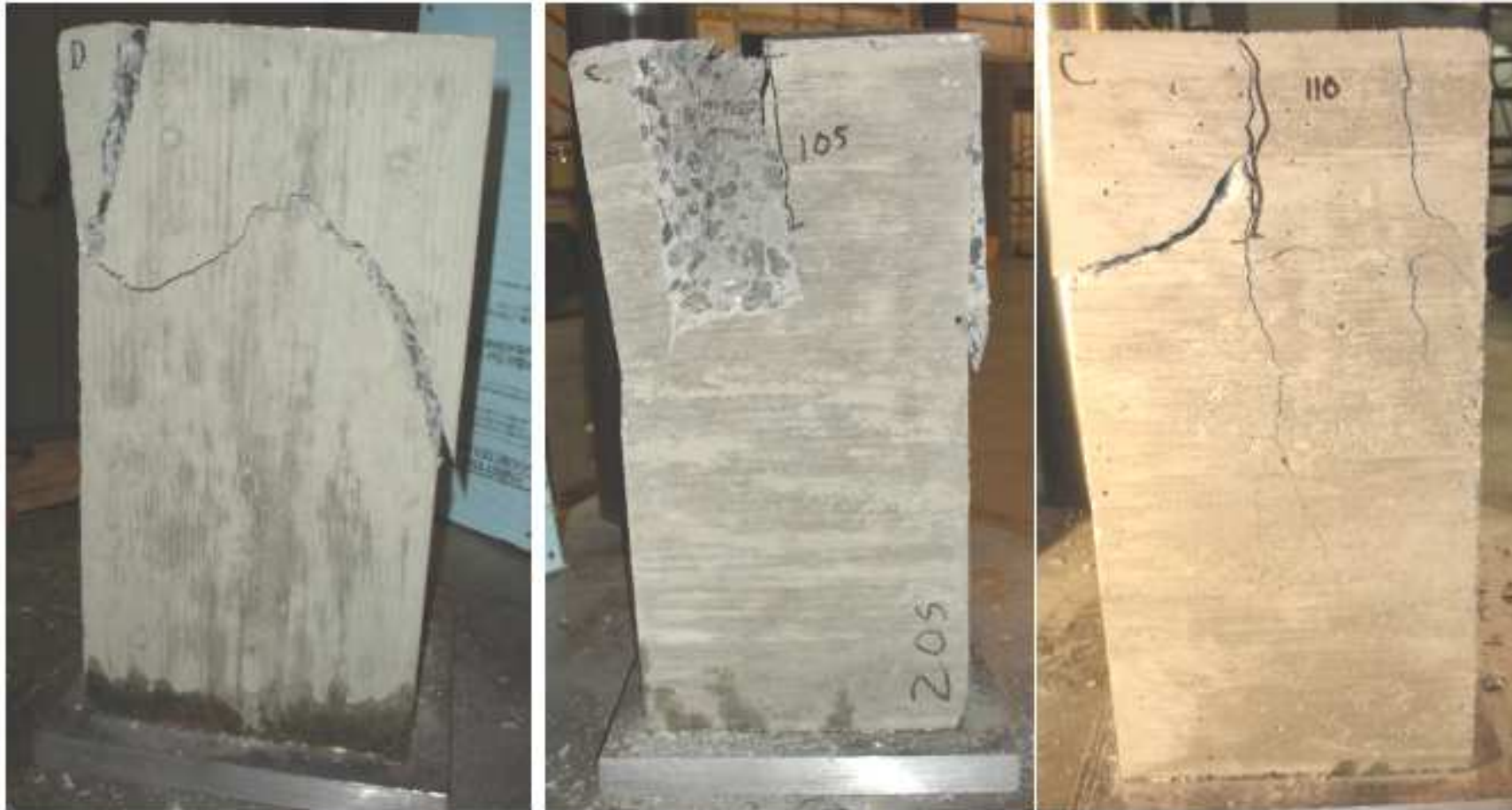
Figure 4-10: Failed Prisms with Spiral Reinforced Prismas com fretagem helicoidal
