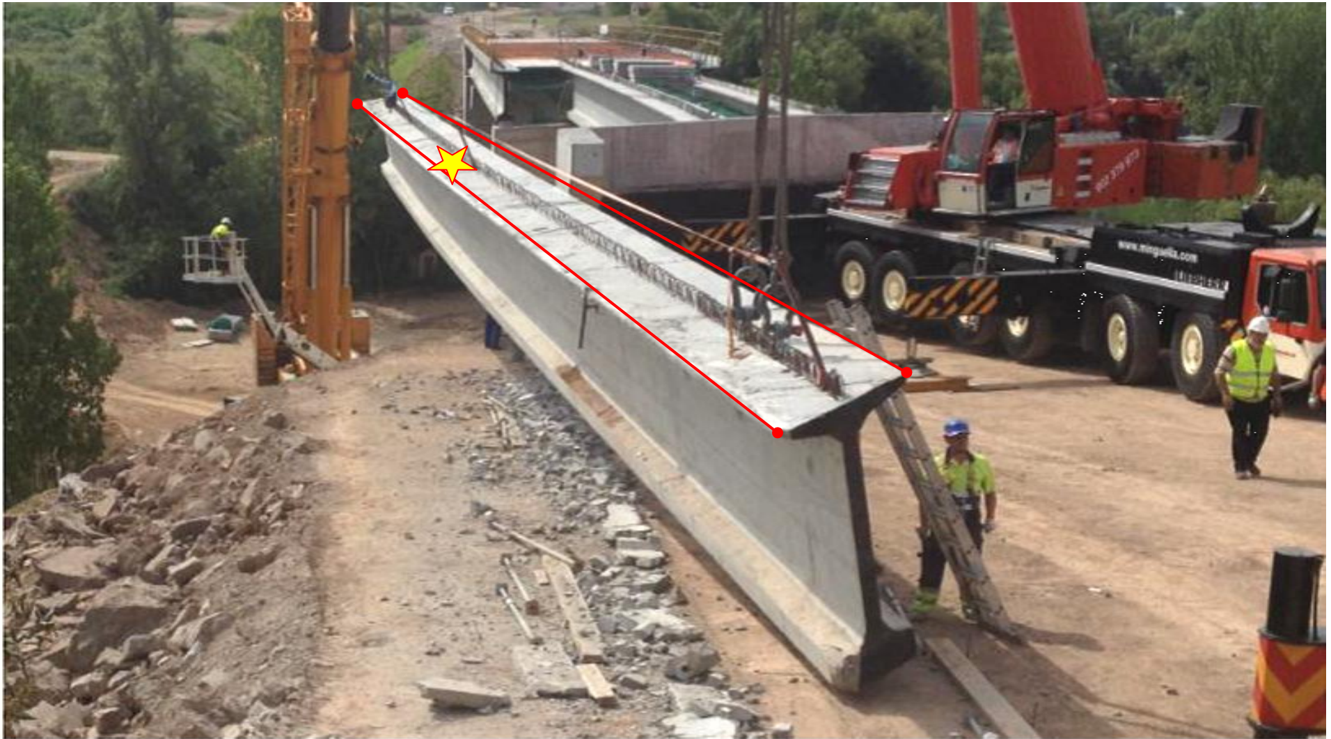
Figure 6.1. Perspective of bridge girder I200B120 during lifting.
