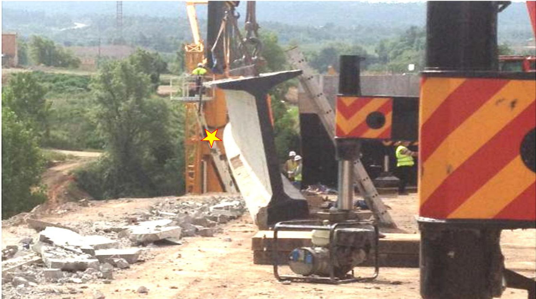
Figure 6.2. Bridge girder I200B120 during lifting.
