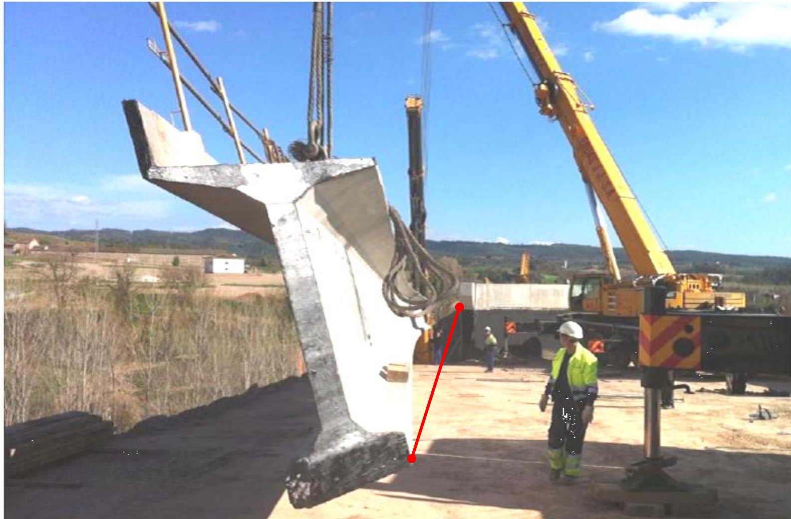
Figure 6.3. Bridge girder I200B120 with modified top flange during lifting.
