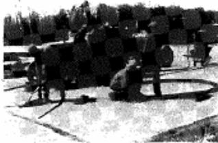
Mud truck raises slabs by forcing mud under them. It consists of a chamber where the mud is mixed, a pump and a pressure hose and is powered with a diesel engine.
