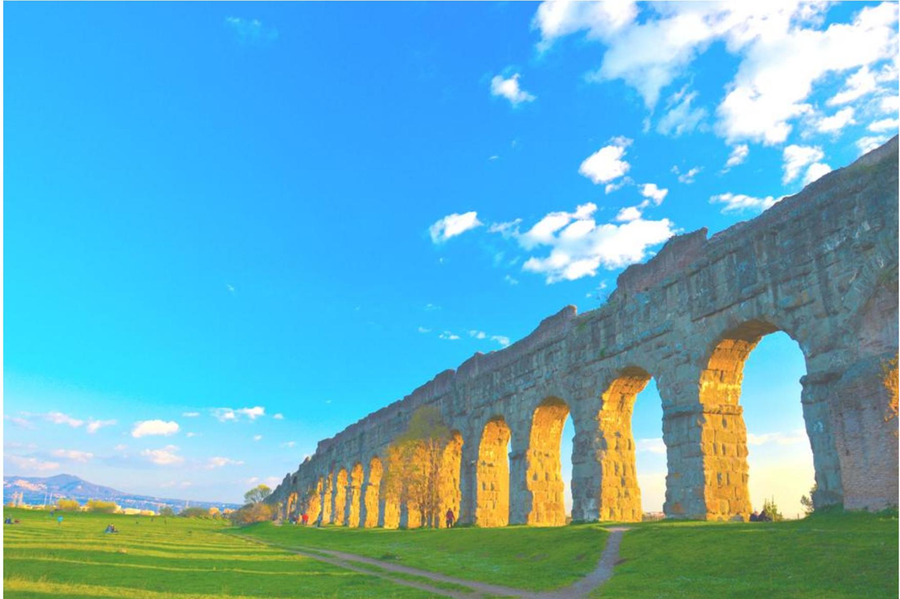
**Aqua Marcia** - Remains of the stone arches and the channel of the Aqua Marcia (140 BC), with the brick Aqua Julia (125 BC) and minor brick remains of the Aqua Tepula (33 BC) on top.
