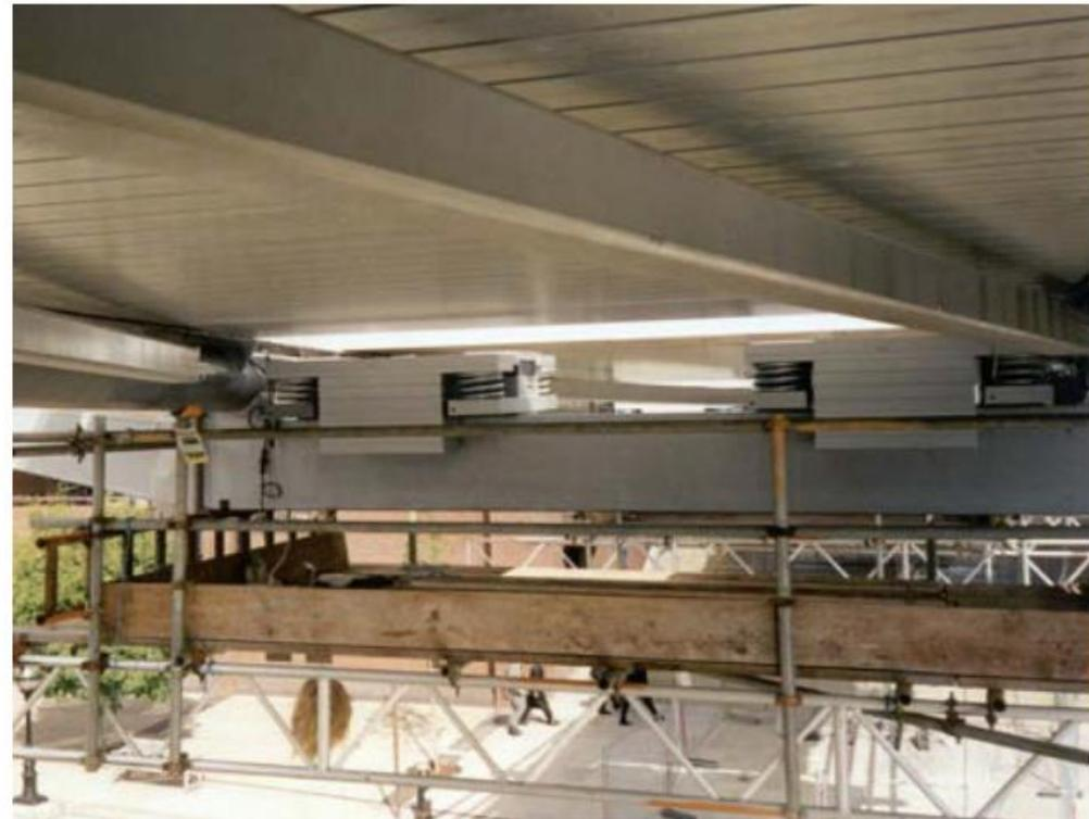
(b) laterally- and (c) vertically-acting tuned-mass absorbers
