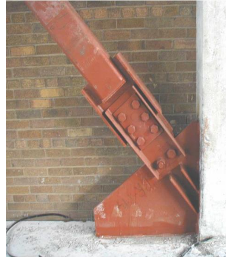
Friction damper in single diagonal bracing
